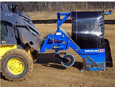
Burchland Silt Fence Installer
